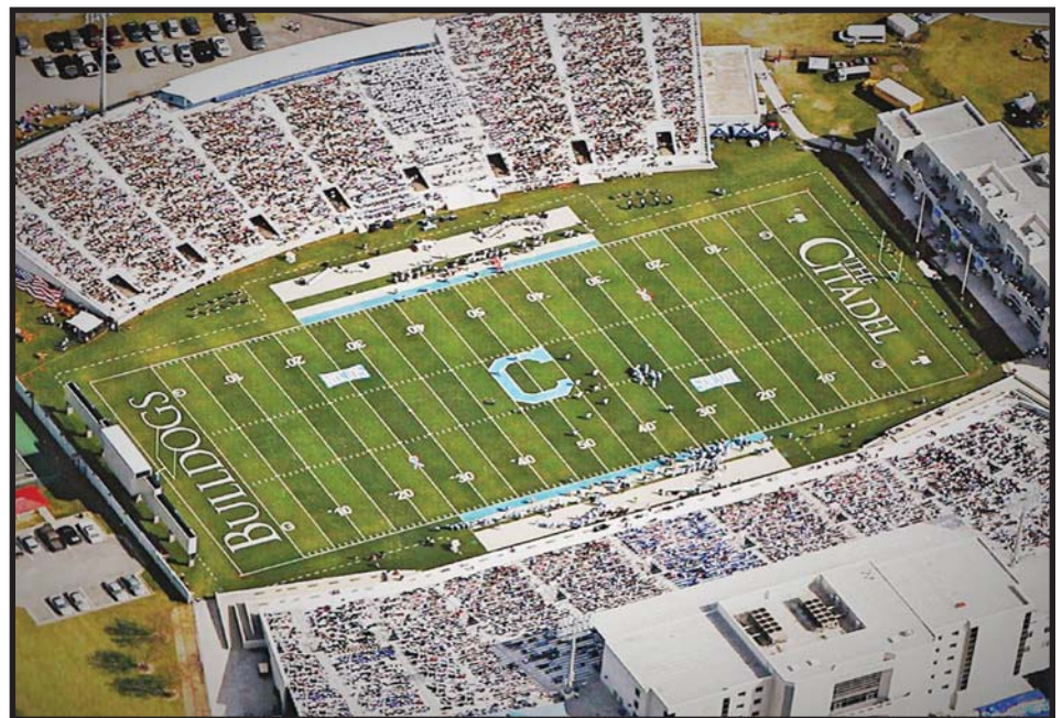
JOHNSON HAGOOD STADIUM (11,332)
